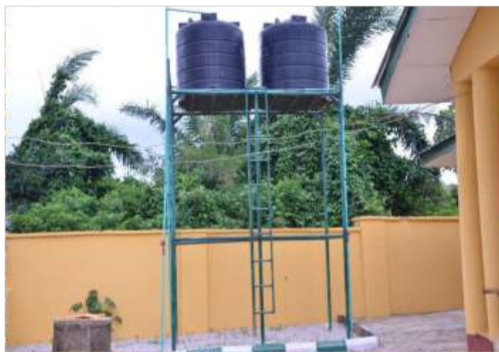
Water storage stand after renovation
